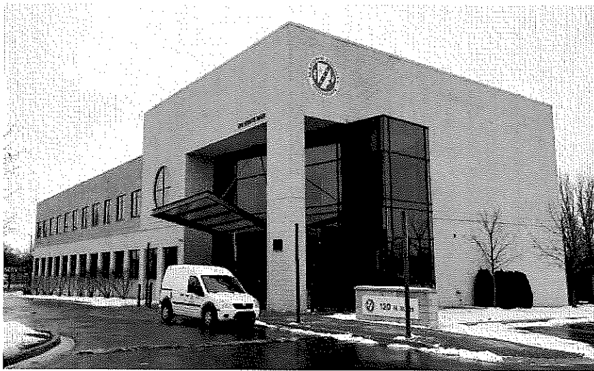
The Talmer building at 120 N. Main in Mount Clemens will house Macomb County offices such as clerk and register of deeds.
