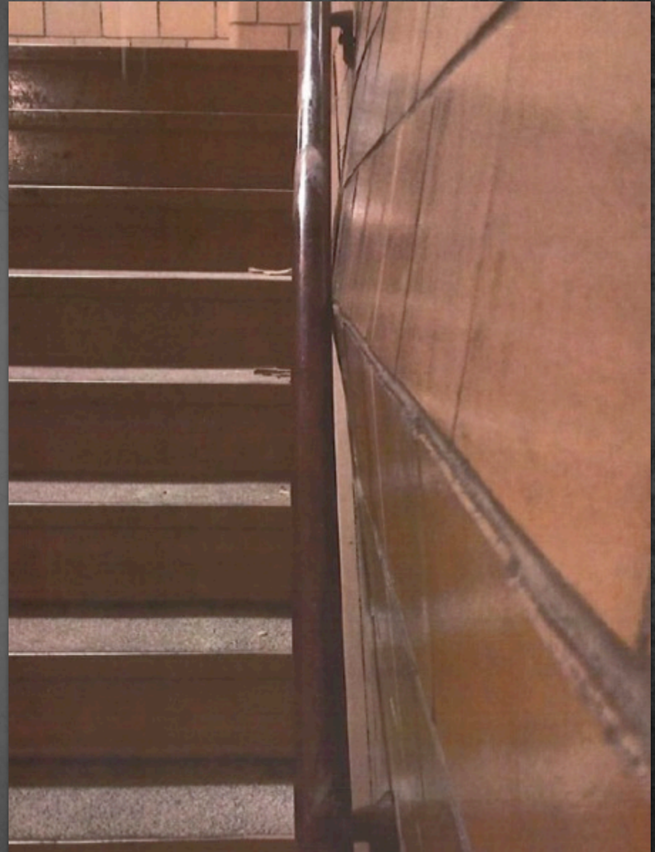
NORTH WALL / NORTH STAIR
