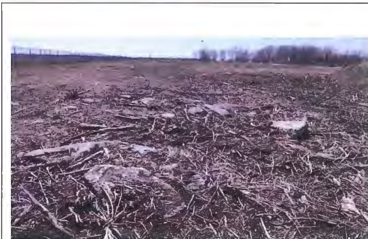
Photo 10. Concrete debris near southeast Property corner
