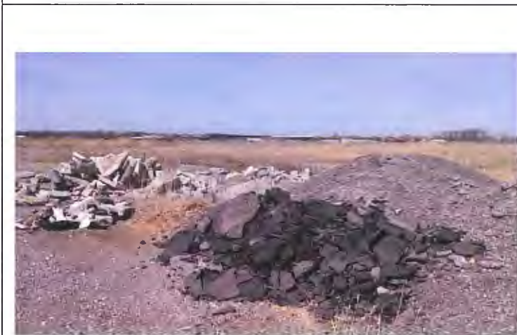
Photo 11. Construction debris on southern area, west of Towne Centre Boulevard
